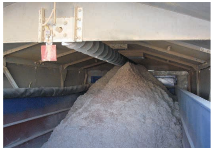
LP baghouse dust collectors can be equipped with bin houses to shelter 40 yard (36.6 m) dumpsters and dust from adverse weather conditions. The bin houses come with ceiling-mounted leveling screws, which evenly distribute dust throughout the entire dumpster.
