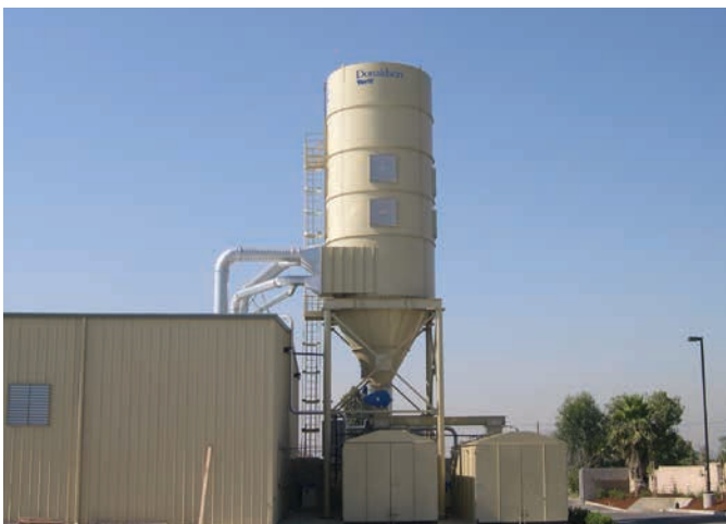
LP baghouse dust collectors can be equipped with bin houses to shelter 40 yard (36.6 m) dumpsters and dust from adverse weather conditions. The bin houses come with ceiling-mounted leveling screws, which evenly distribute dust throughout the entire dumpster.
